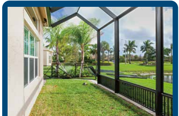
Construction Screen Installation
